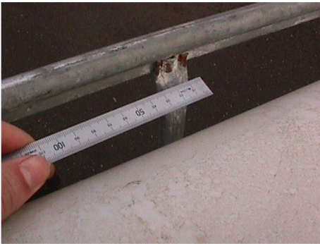
Pic 4: Rust is less than 25mm (1 inch) - acceptable
