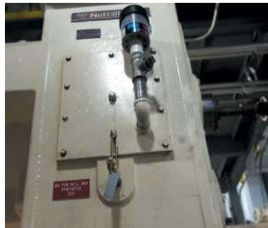
Sight glass added with oil sample port combo. Desiccant breather with stainless piping and top-off plug between gearbox and breather.
